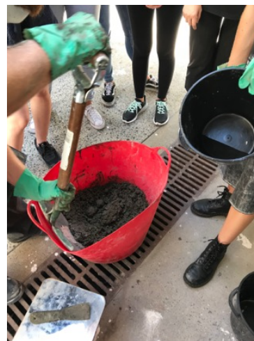
Image 3: Mixing concrete with shovel
