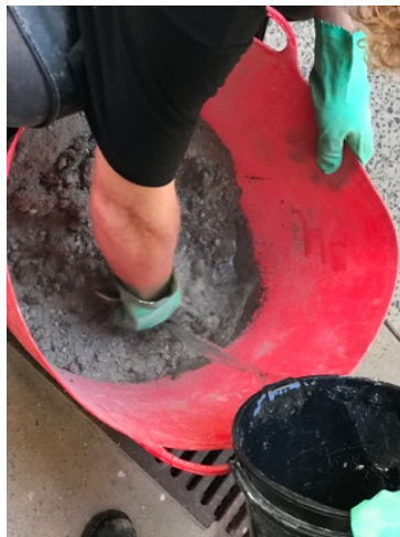
Image 2: Adding water into concrete
