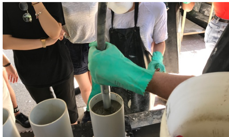
Image 5: Using concrete vibrator to even out concrete
